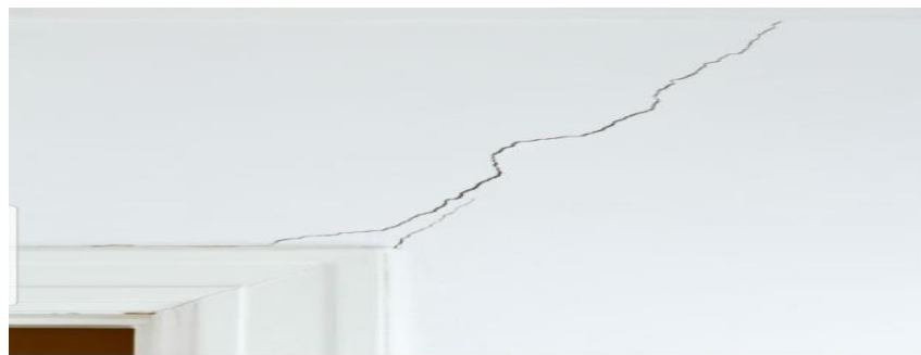
Fig. 2: shows the cracks at the top of the window
