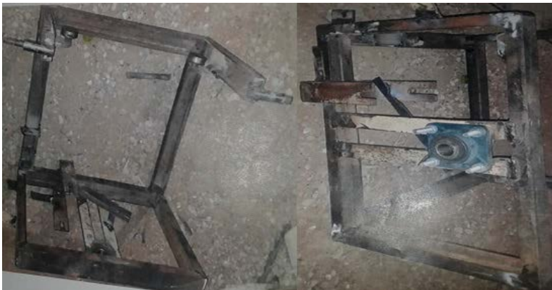
Figure 3: Fabrication of concrete mixer body.
