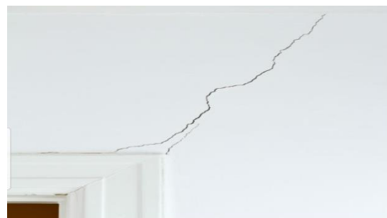
Fig. 3: shows the cracks at the top of the window
