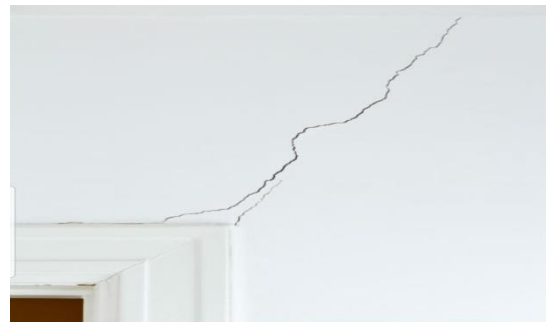
Fig. 2: shows the cracks at the top of the window
