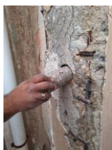
Fig. (17): Extracting concrete core
