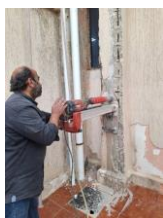
Fig. (16): One of the places where drilling concrete cores are extracted
