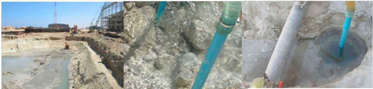
Figure 2. well points in (Zhou Benghazi tower).
