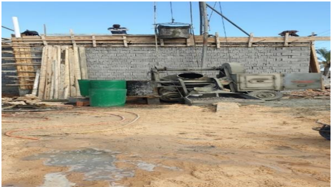
Figure 11 manual machine mixing and pouring
