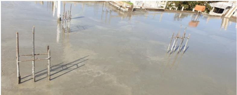
Figure 10 increasing water for concrete in the upper layer
