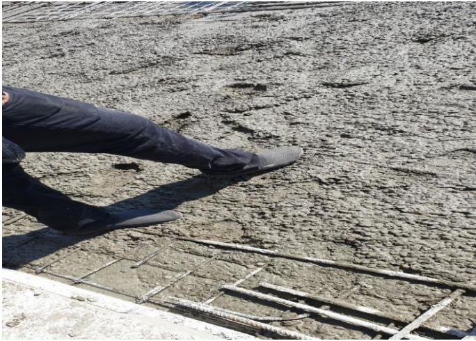
Figure 12 delayed pouring of the second layer
