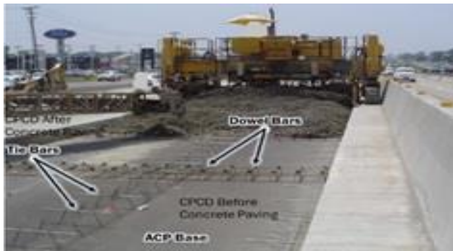
Fig. 8: Concrete Pavement Contraction [26]
