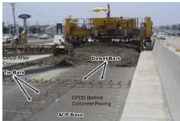
Fig. 7: Continuously Reinforced Concrete Pavement [21]
