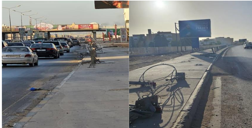
Figure (4): Damaged Safety Barriers
