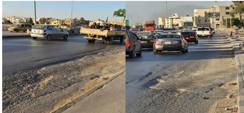
Figure (3): Road Surface Defects
