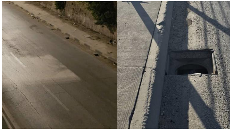
Figure (2): Uncovered Stormwater Drain Openings
