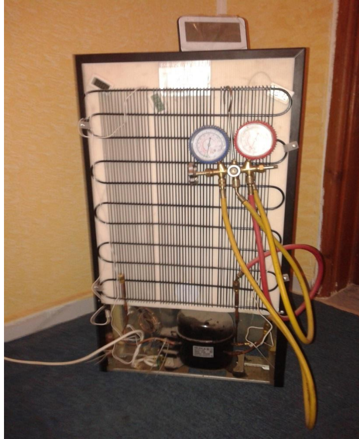
Figure (2) Installation of pressure and temperature measuring devices for a home refrigerator
